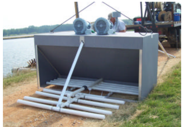
The RELIANT Model WQA dual blower, dual diffuser Water Quality and Aeration System being installed in a catfish pond.
